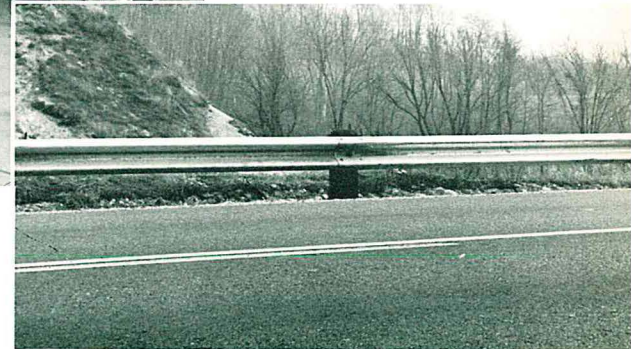
A galvanized guard rail lining an Indiana highway.
