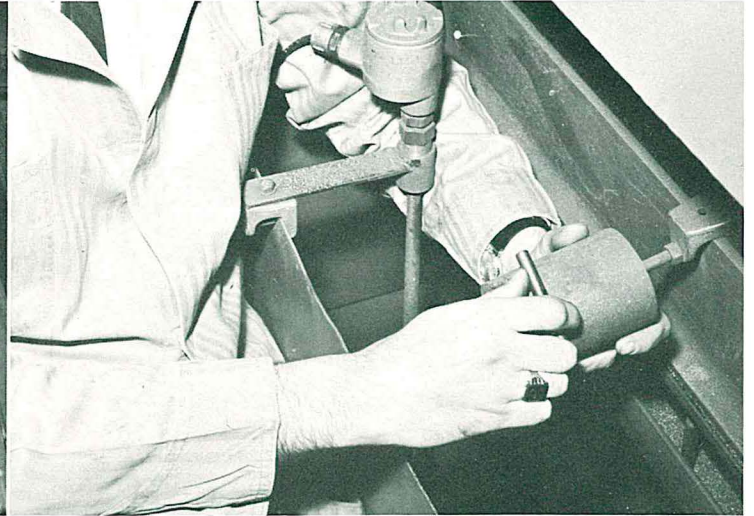
Adjusting the abrasive separator assures that only sound, effective abrasive is used.
